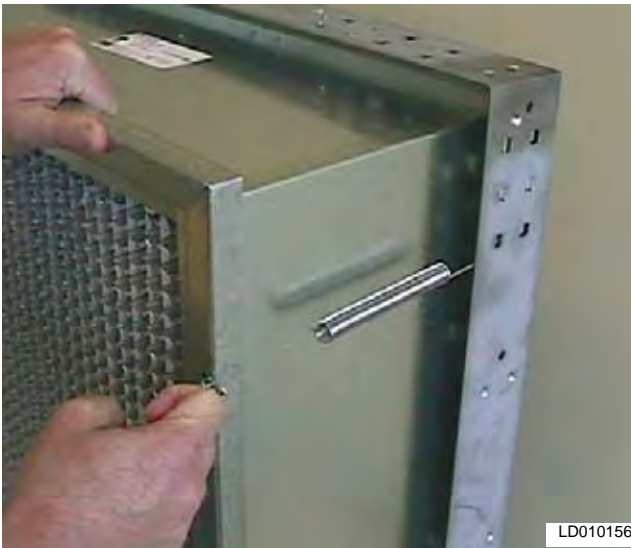
FIG. 4-33 – FRAME WITH 4 LATCHES INSTALLED
