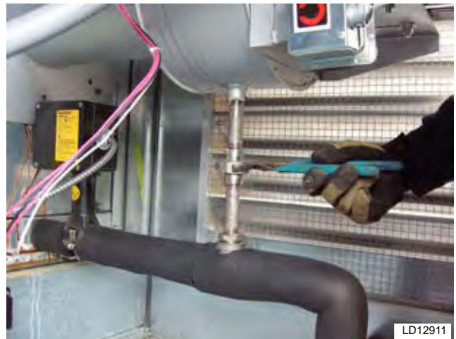
FIG. 3-20 – CONDENSATE DRAIN
