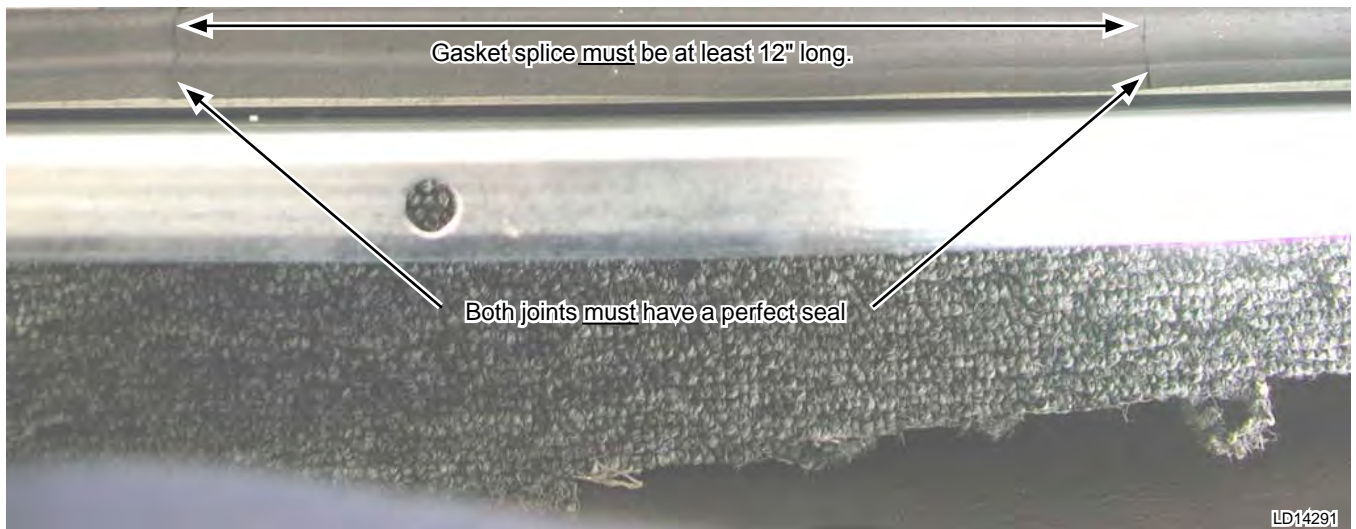
FIG. 5-86 – GASKET SPLICE REQUIREMENTS
