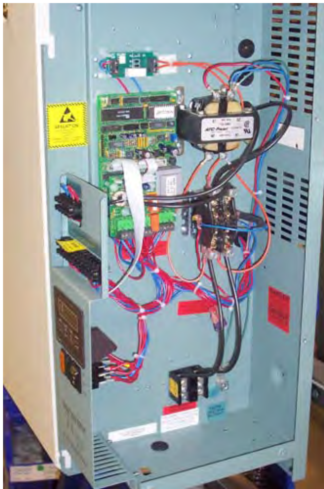
FIG. 2-62 – TYPICAL HUMIDIFIER PANEL LAYOUT
