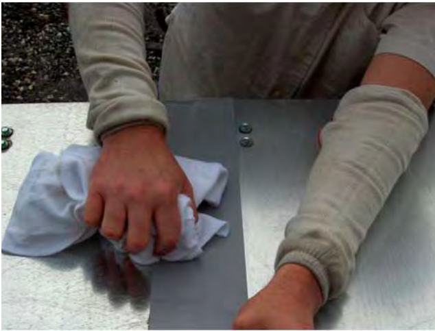
FIG. 5-97 – APPLY PRESSURE - ROLLER RECOMMENDED
