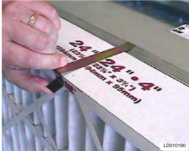
FIG. 4-36 – SPRING THE END OF THE LATCH SO THAT IT FITS OVER THE EDGE OF THE PREFILTER. (4" W/315-003-004 LATCH SHOWN)
