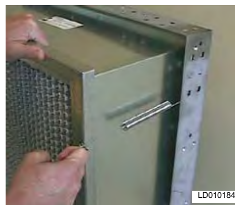
FIG. 2-109 – SPRING LATCH SHOULD BE PULLED AND FASTENED IN HOLE IN THE HEADER OF THE FILTER.
