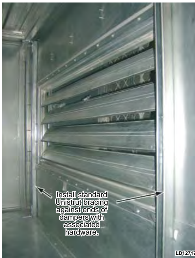
FIG. 5-121 – INSTALL BRACING TO MIXING DAMPER WALL ON EITHER SIDE OF DAMPERS
