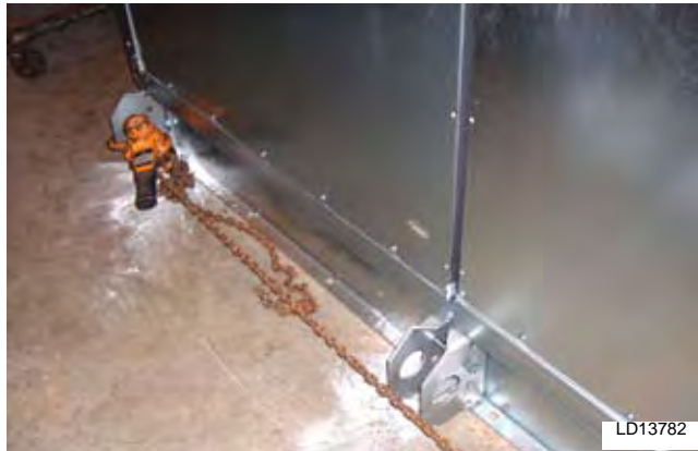
FIG. 2-25 – PLACING & ANCHORING FIRST SECTION AND ATTACHING COME-A-LONGS
