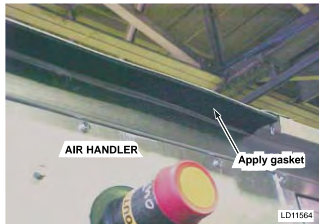
FIG. 2-41 – INSTALL GASKET UNDER ROOF OVERHANG
