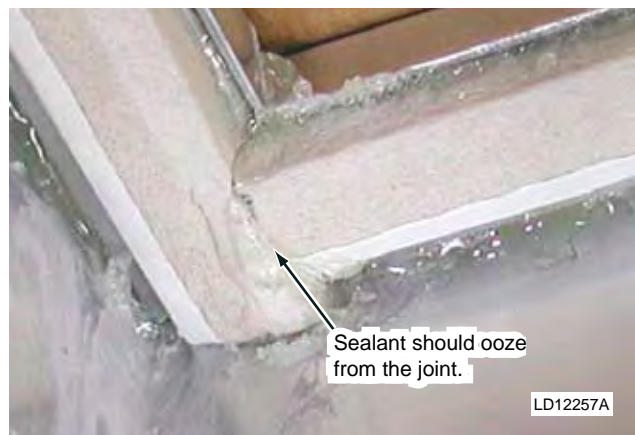
FIG. 5-54 – GOOD VERTICAL TO HORIZONTAL BUT JOINT
