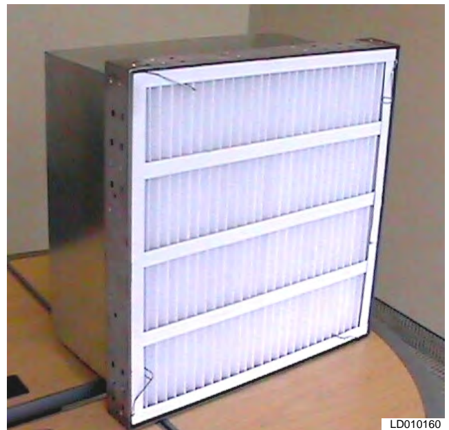
FIG. 4-27 – FULLY INSTALLED FILTERS
