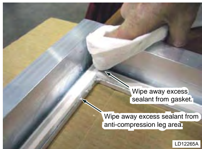
FIG. 5-62 – WIPE OFF EXCESS SEALANT
