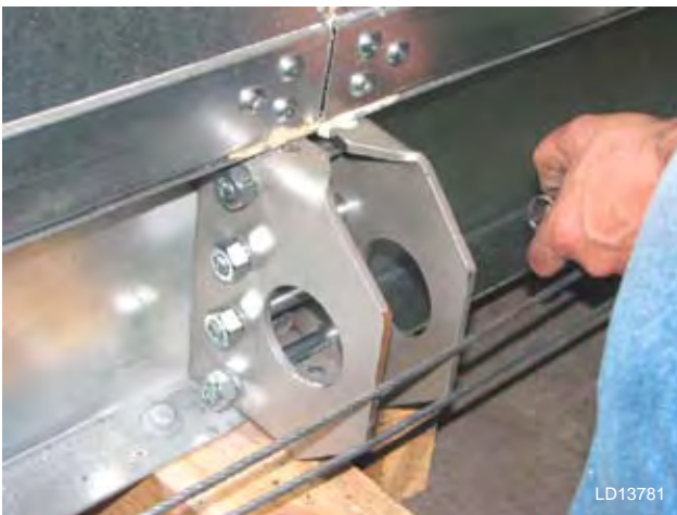
FIG. 2-28 – INSTALLING BOLTS AFTER PULLING UNITS TIGHT TOGETHER
