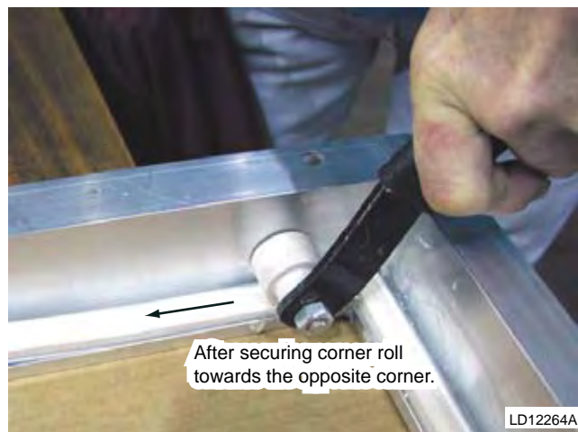
FIG. 5-61 – ROLL TOWARDS OPPOSITE END OF VERTICAL GASKET
