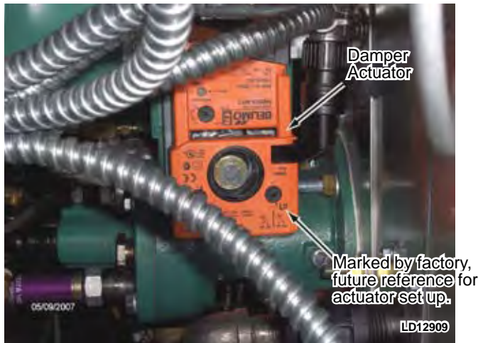
FIG. 3-19 – DAMPER ACTUATOR
