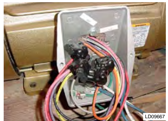
FIG. 5-23 – MOTOR WIRE CONNECTIONS
