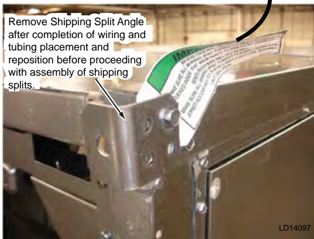
FIG. 2-19 – REMOVE AND REPOSITION SHIPPING SPLIT ANGLE
