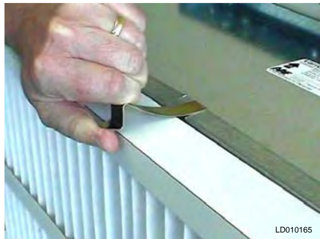
FIG. 4-35 – POSITION PREFILTER IN FRONT OF THE FINAL FILTER. (2" W/315-003-002 LATCH SHOWN)
