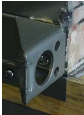
Raceway Lifting Lug (at shipping split)
