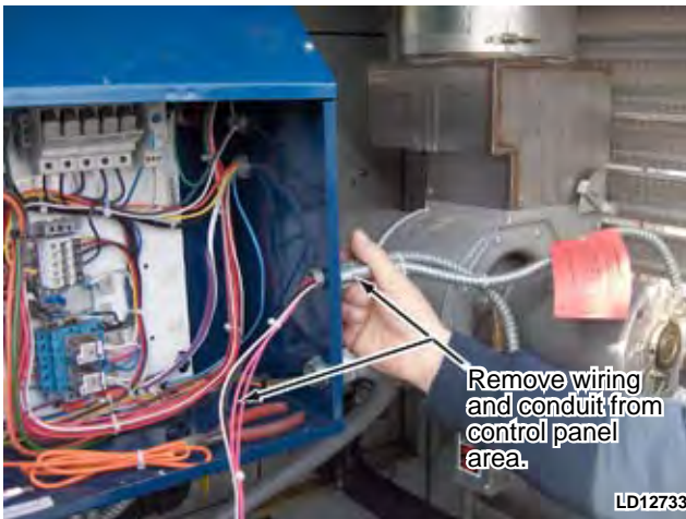
FIG. 5-127 – REMOVE WIRING AND CONDUIT FROM CONTROL PANEL
