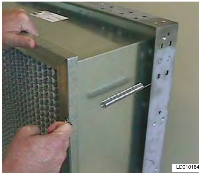
FIG. 4-31 – SPRING LATCH SHOULD BE PULLED AND FASTENED IN HOLE IN THE HEADER OF THE FILTER.
