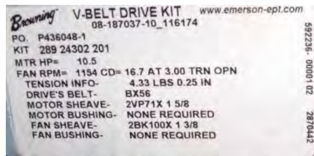
FIG. 3-8 – TYPICAL DRIVE KIT DATA TAG
