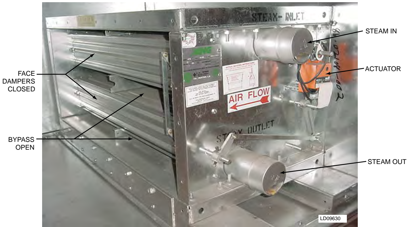
FIG. 2-72 – INTEGRAL FACE & BYPASS COIL (HORIZONTAL; TUBES, STEAM SHOWN)
