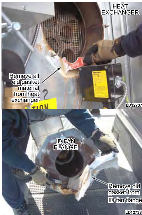
FIG. 5-132 – REMOVE OLD GASKET
