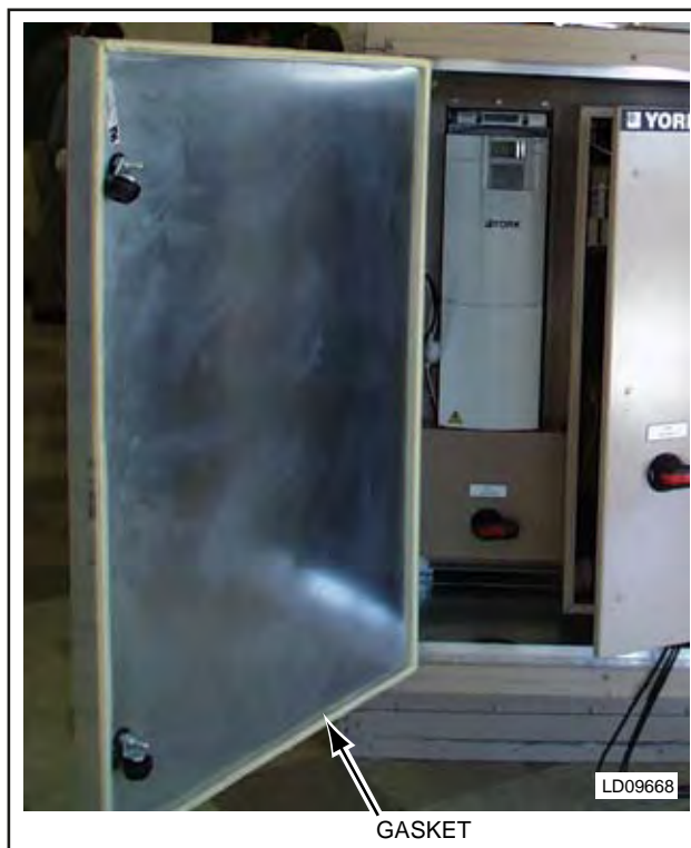
FIG. 5-26 – OLD STYLE DOOR WITH MITERED CORNER GASKET
