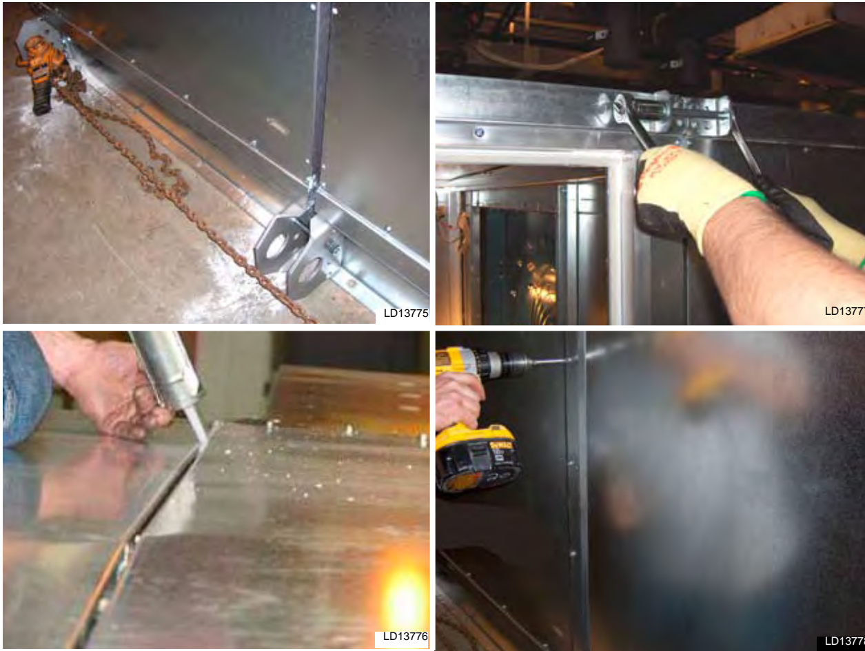
FIG. 2-20 – BRINGING SECTIONS TOGETHER
