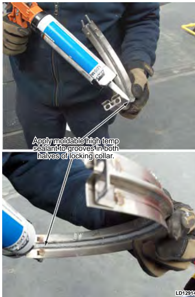
FIG. 5-137 – APPLY SEALANT TO LOCKING COLLAR GROOVES
