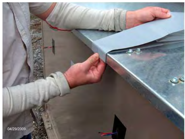
FIG. 5-95 – UNDER DRIP AND OVERHANG
