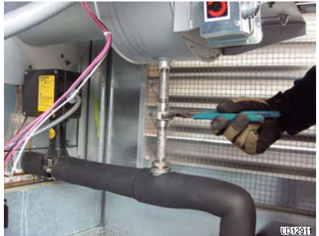
FIG. 3-19 – CONDENSATE DRAIN
