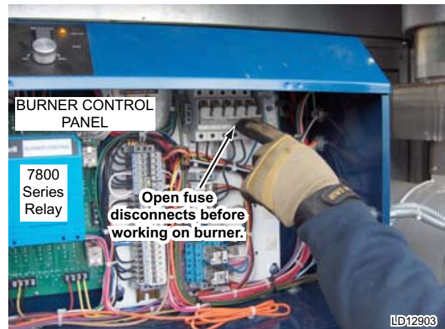
FIG. 3-13 – OPEN FUSE DISCONNECTS
