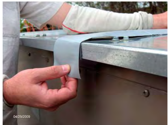
FIG. 5-94 – APPLY CENTERED OVER SEAM
