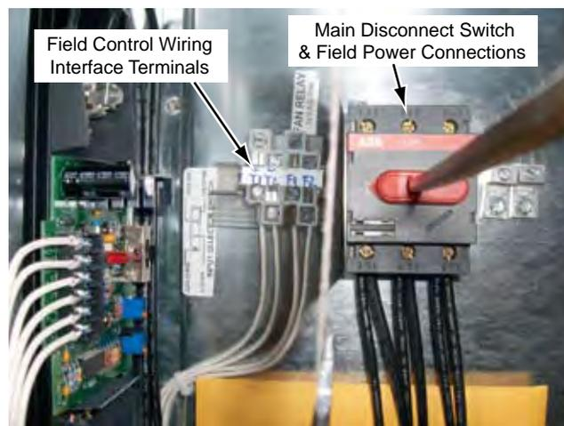
**FIG. 2-59 – TYPICAL FIELD CONTROL AND POWER CONNECTIONS**
