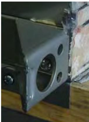
**Raceway Lifting Lug (at shipping split)**
