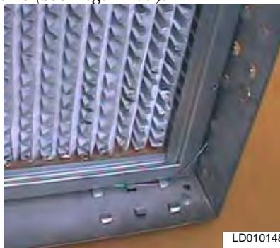
**FIG. 2-103 – INSTALLED CARTRIDGE FILTER**
