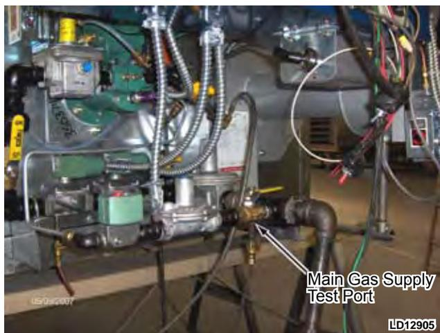
**FIG. 3-16 – CHECK MAIN GAS SUPPLY PRESSURE**
