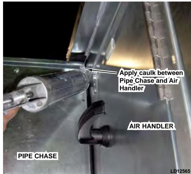
FIG. 2-47 – PIPE CHASE TO AIR HANDLER CAULK APPLICATION
