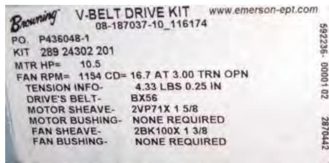
FIG. 3-8 – TYPICAL DRIVE KIT DATA TAG
